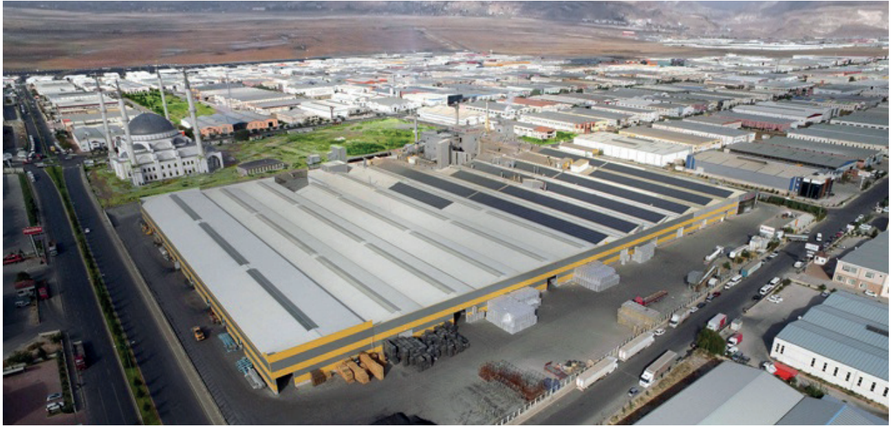
RAVABER Kayseri Manufacturing Plant, Turkey
