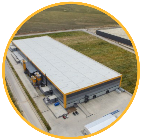
ODE Eskişehir, Turkey Production Facilities
